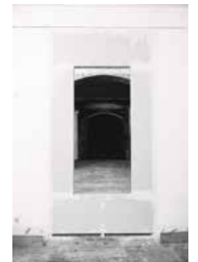
and four plaster boards seal the doorway.
