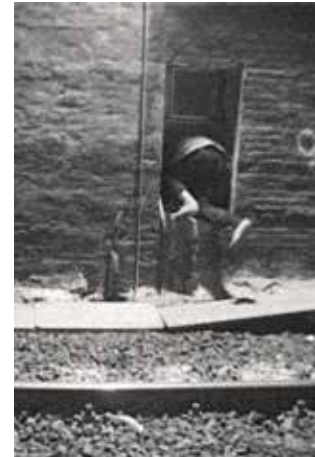
Temporary cut-out passageway.
