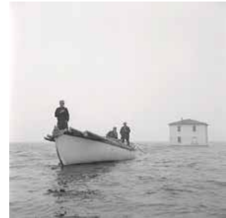
A house, buoyed with oil-drums, relocating along the coast of Newfoundland, Canada.
