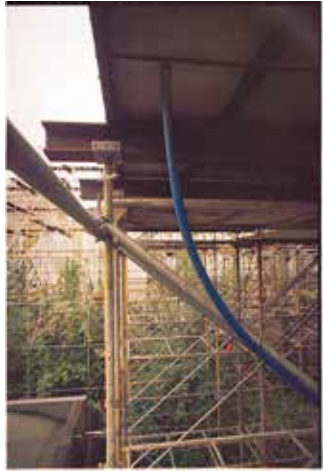
Snaking soil pipe.
