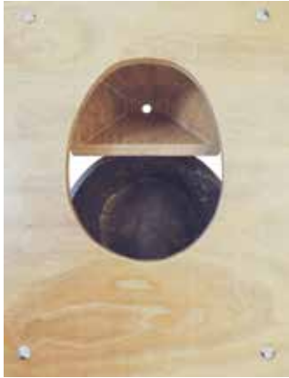
The separating toilet.
