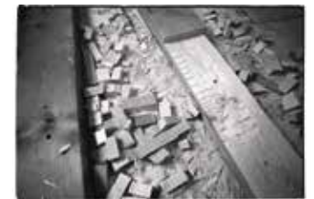
Soon-to-be support beams for the roof structure, with cut-out slots for the sliding windows.
